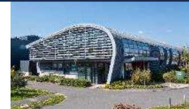
Aerospace Technology Centre Industry collaboration/co-location
