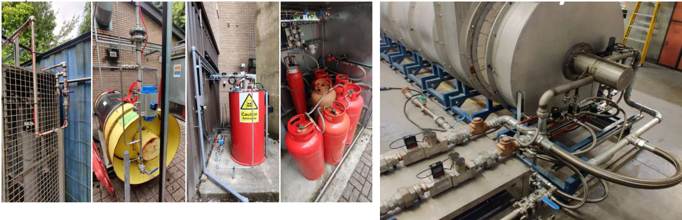
Automatic ammonia-hydrogen ( NH_3/H_2 ) combustion system
